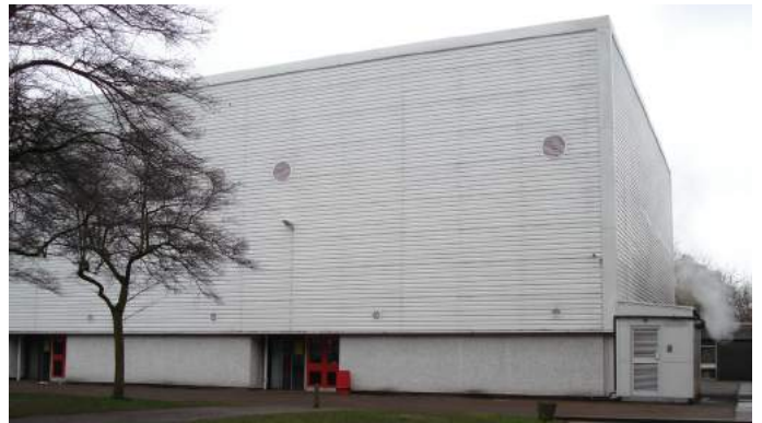
Recent overcladding of swimming pool & gymnasium building
