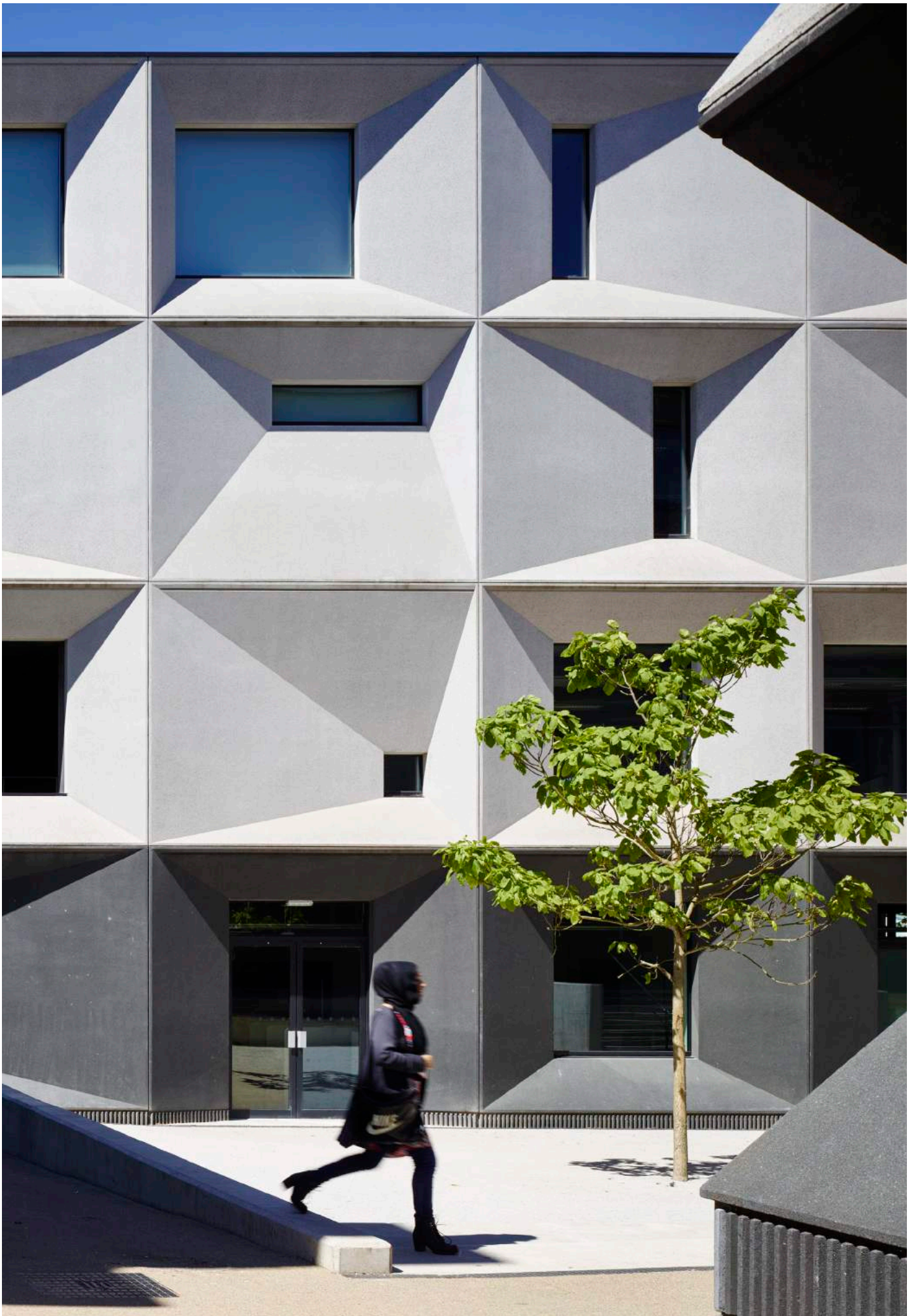
Detail of precast faceted concrete façade panels
