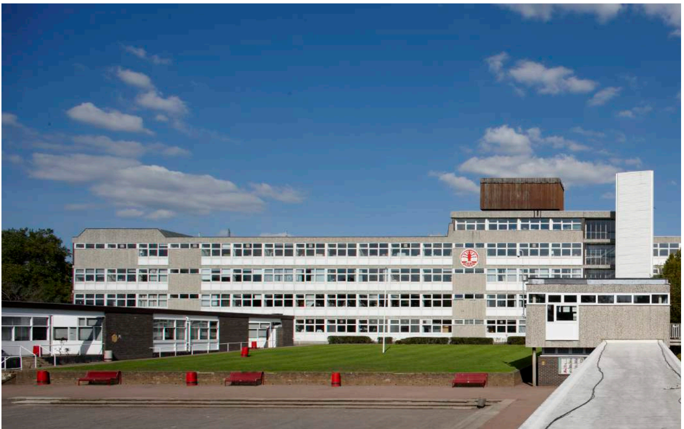
Existing Burntwood School campus
